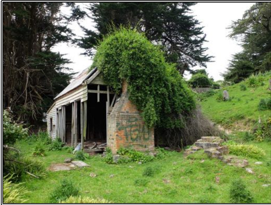
Figure 56 Stewart's house, with the brick foundations of another building in the right foreground.
