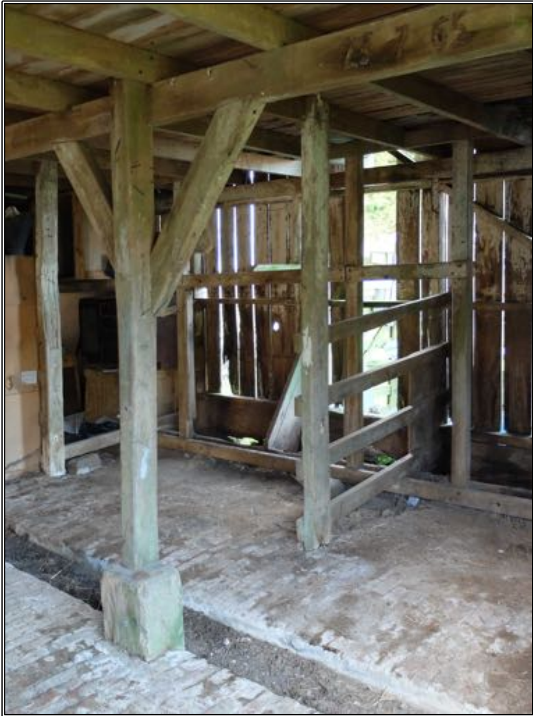
Figure 187 The most intact and unmodified section of stalls within the byre (on the east side of the building), showing the main internal braced post, the effluent drain, the stall railings and the mangers. The remnants of whitewashing can also be seen.
