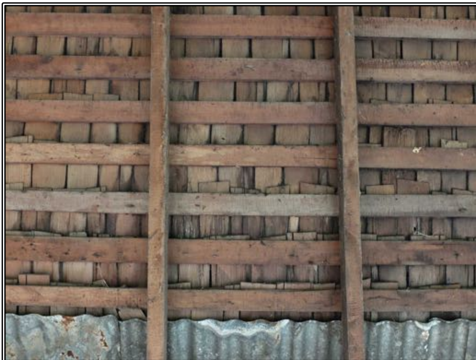
Figure 208 A detail of the rafters, purlins and shingles in the roof structure. All timber shown here were pit-sawn or axe-split.
