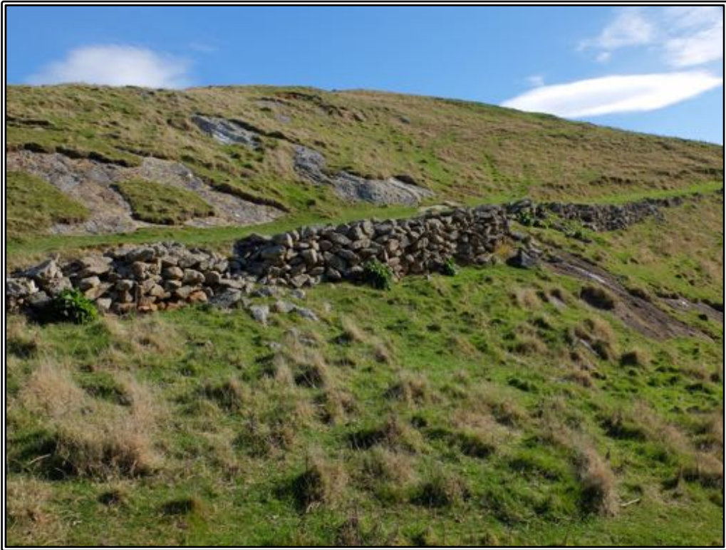
Figure 93 Stone revetment on Rutherford's Road east (I44/423)
