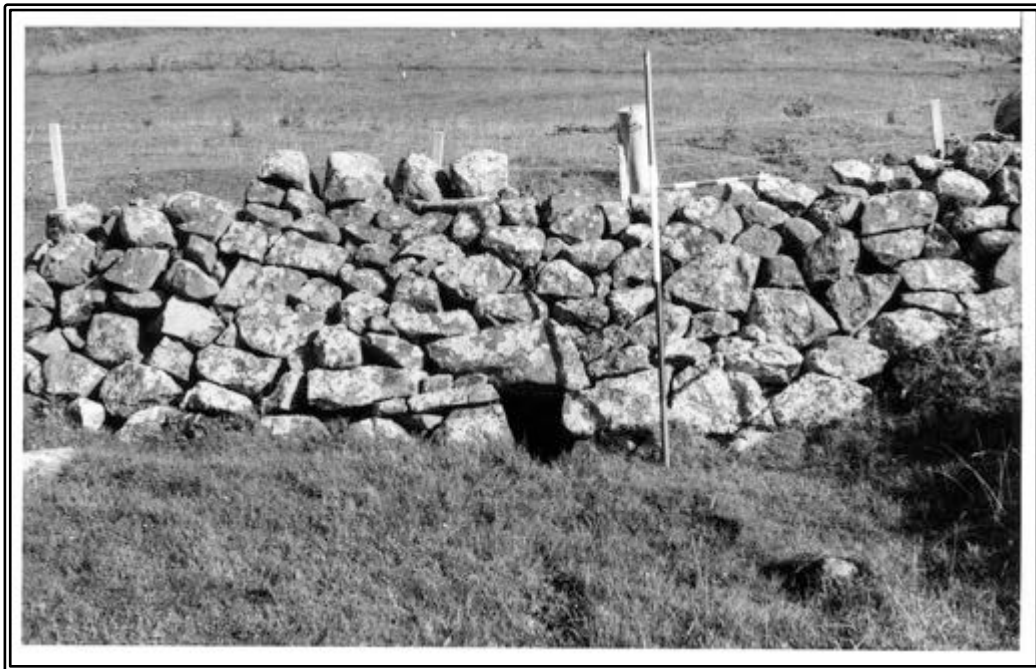
Figure 6 Stone wall I44/410: Wall 21A illustrated in Higham 1986, showing a water smoot through the wall.
