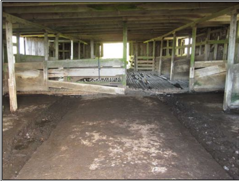
Figure 162 The sheep pens half way through being removed in 2017, exposing the original floors and pens.
