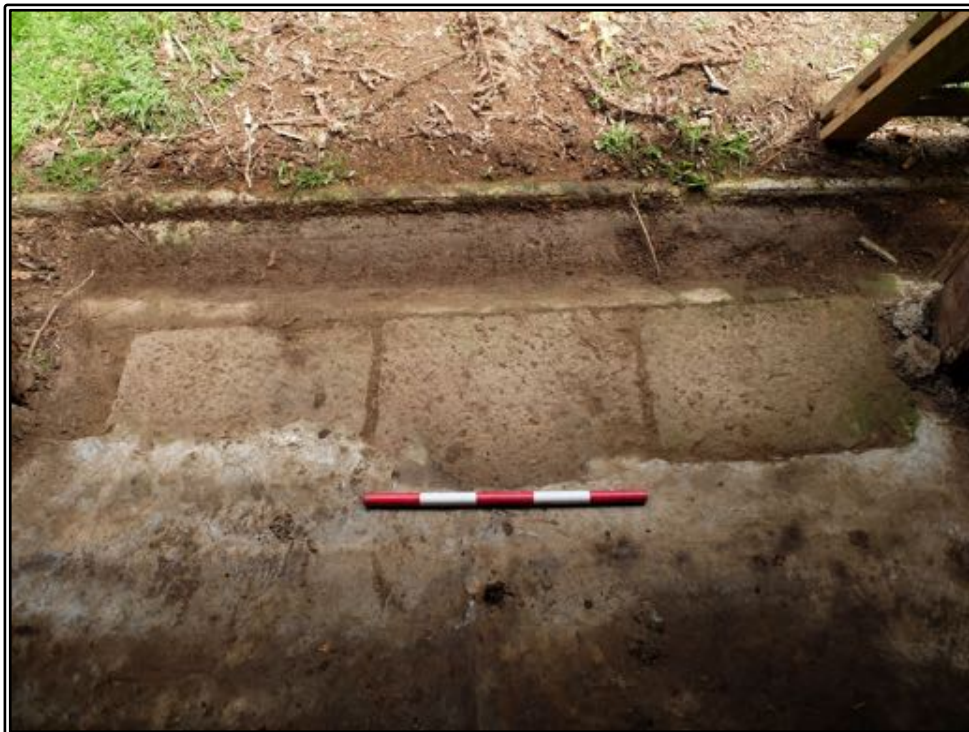
Figure 165 Dressed stone paving blocks at the western entrance to Larnach's byre.
