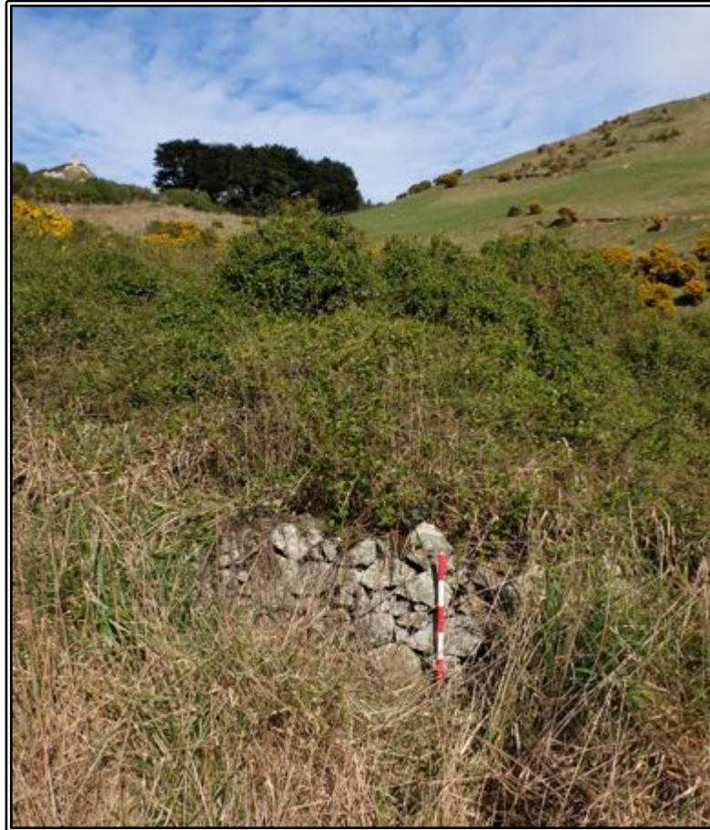
Figure 11 Stone wall I44/411 on the west side of Camp Road.
