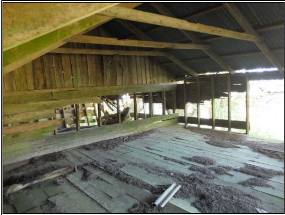
Figure 181 The upper storey in the central area of Riddell's farm building.
