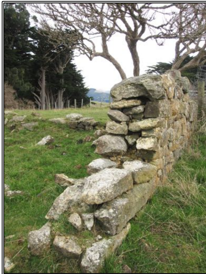
Figure 104 Detail view of the end wall of Nyhon's byre (I44/429), showing how the wall was constructed.
