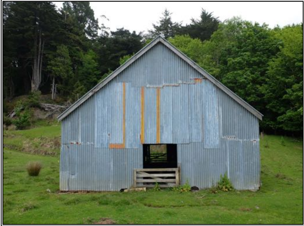
Figure 158 The east wall of Larnach's byre.
