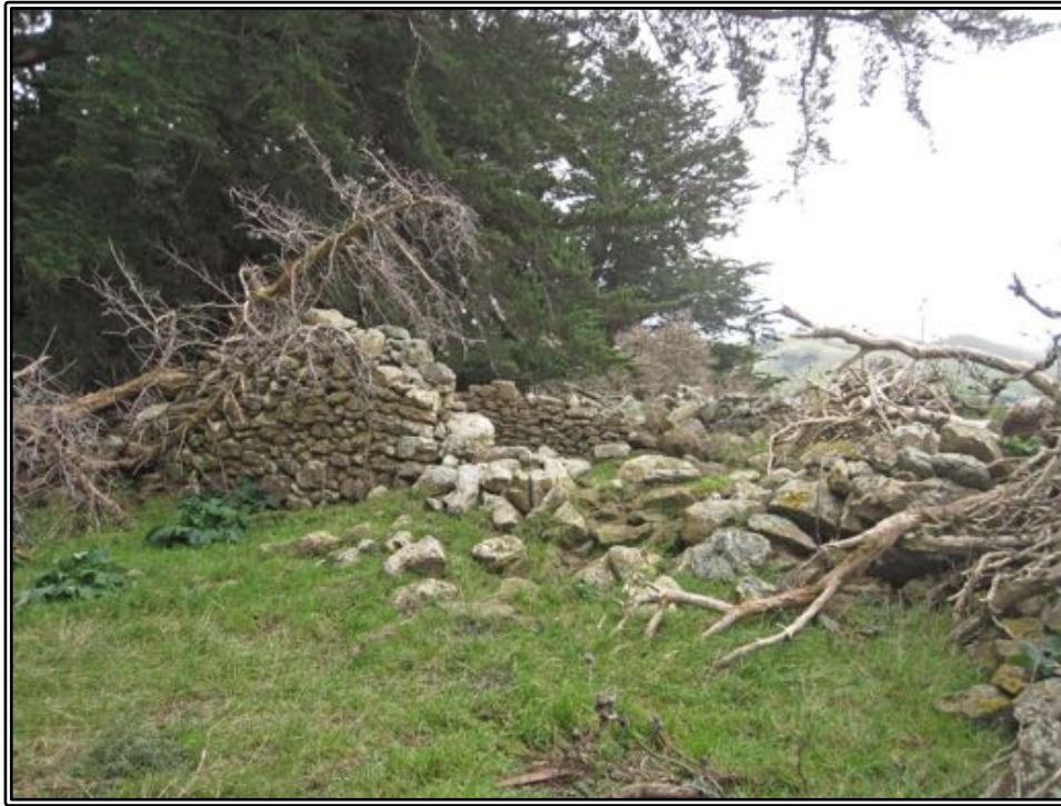
Figure 88 The ruins of the stone farm buildings, on the east side of the main macrocarpa enclosure at Rutherford's farm (I44/426).
