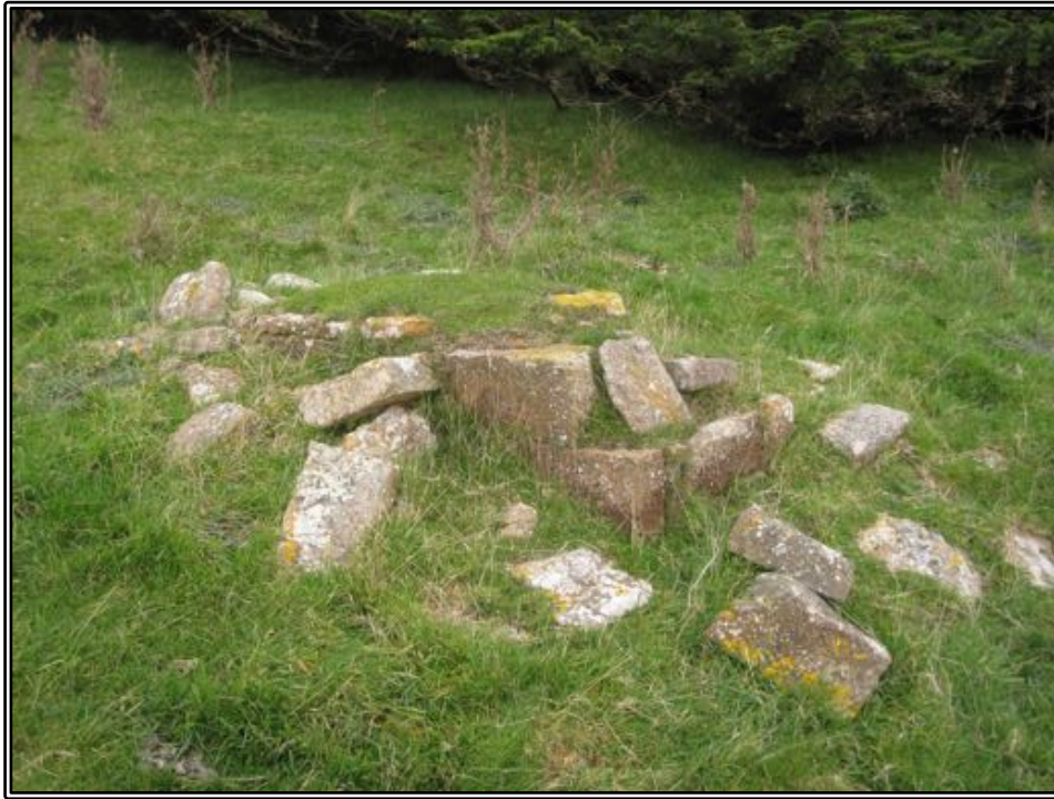
Figure 108 The masonry chimney base at Dick's farmstead (I44/431).
