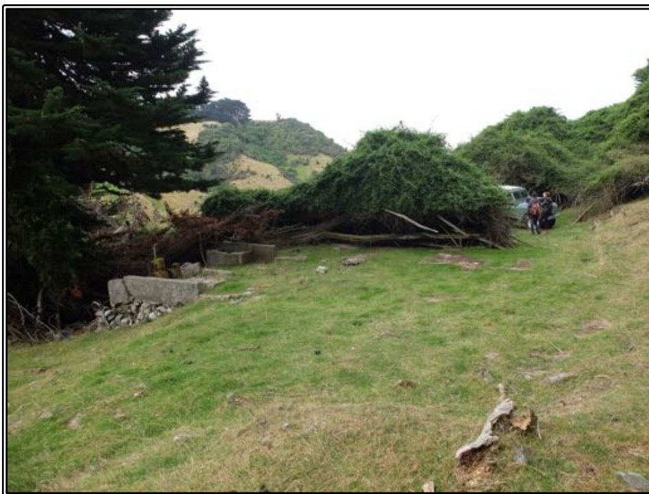
Figure 57 The site of Stewarts byre or cowshed, with the concrete floor and foundations of the engine room to the left.
