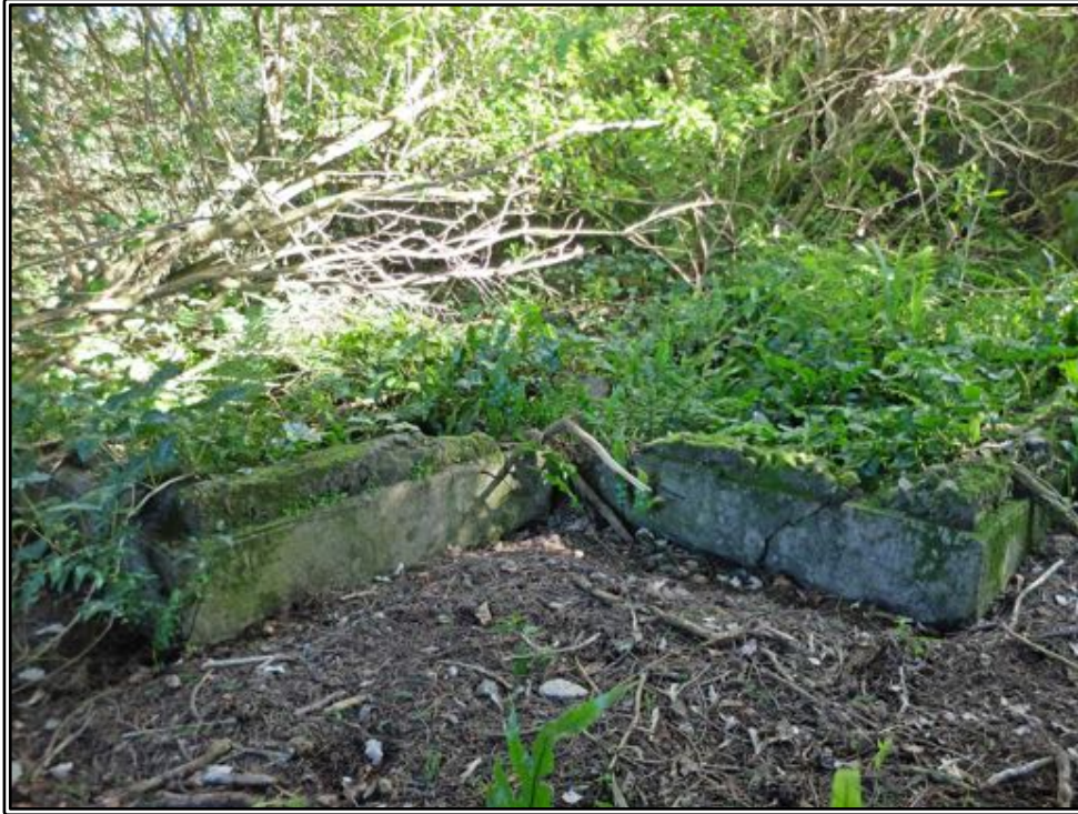
Figure 36 Concrete foundations of Riddell's house.
