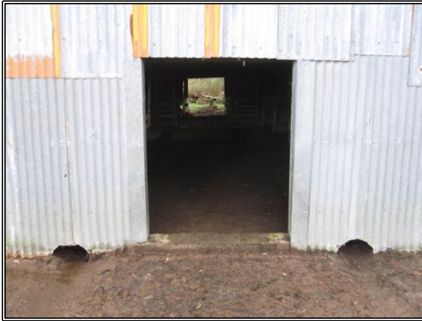
Figure 160 The drain exits cut into the eastern end wall of Larnach's byre, together with the cobbles outside the entrance.
