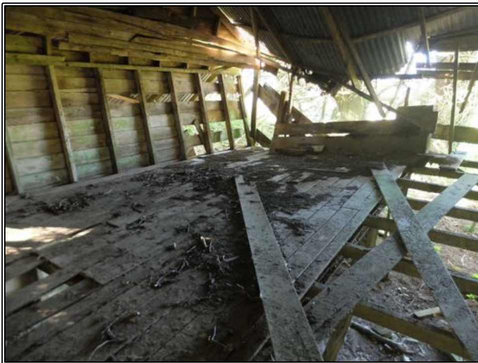
Figure 180 The upper storey at the north end of Riddell's farm building.
